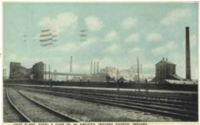
COAL PLANT, STEEL & TUBE CO. OF AMERICA, INDIANA HARBOR, INDIANA.
