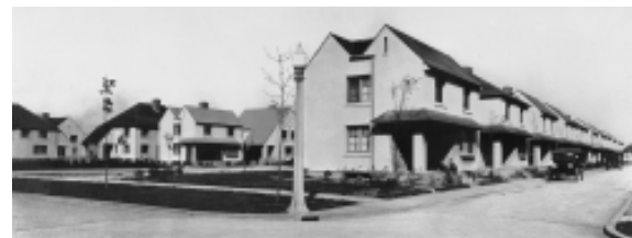
PHASE 1: 1917 Worker Homes
