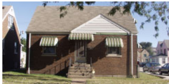
PHASE 2: 1942 brick 4-square (19)
